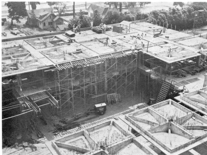
**PROGRESS PHOTO**—In this unique photo, taken from the TOP of the huge crane at the construction site, you can see the massive concrete umbrellas beginning to form the roof of Ambassador's new Dining Hall.
